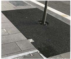
Filter Pave Porous Paving 40mm depth -Starlight Black Colour
