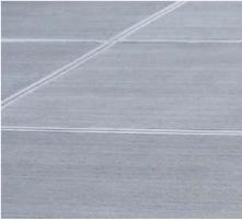
In-situ Concrete - Broom Finish - Natural Grey Colour (No Oxide Colour)
